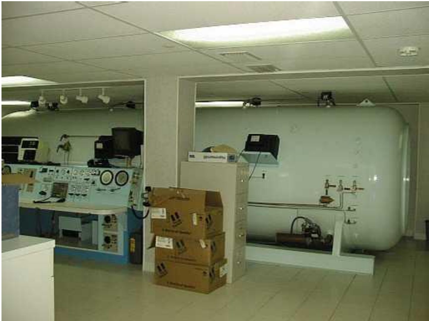
Main Lock End of Chamber
