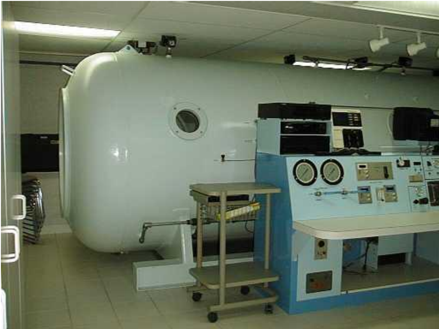
Entry Lock End of Chamber
