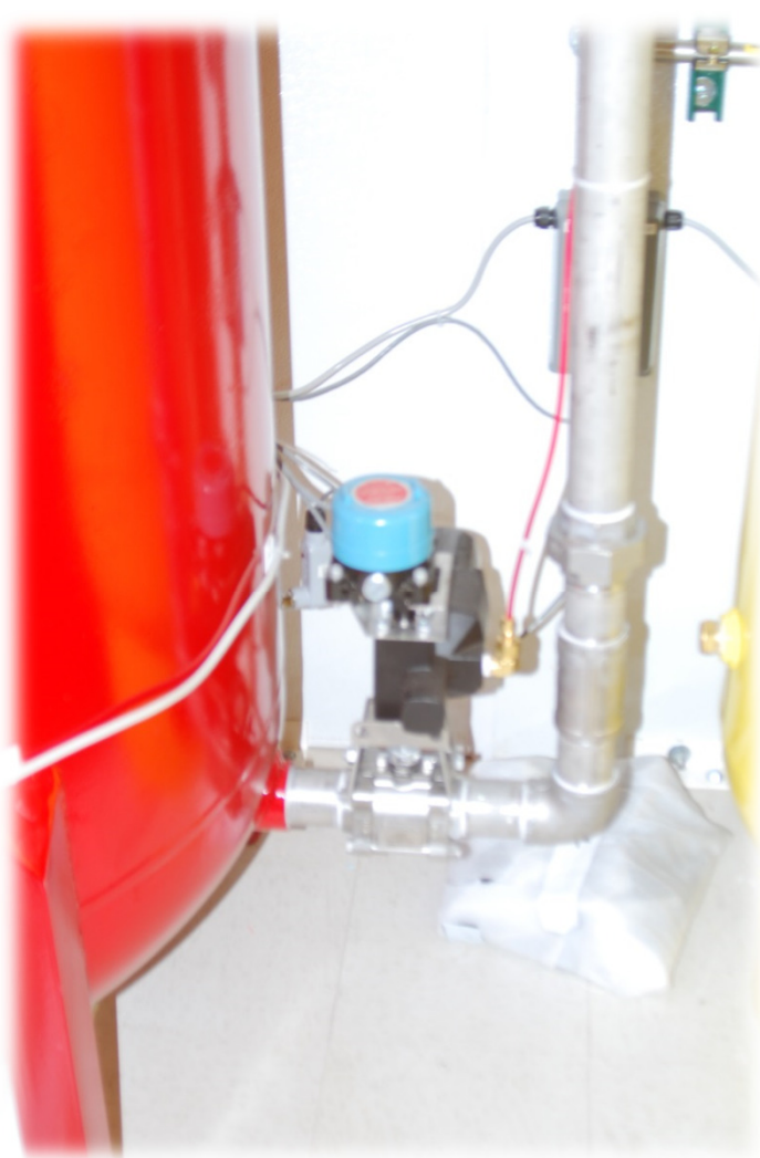
Partial views of FSS Deluge water tank with actuation controls, Air Accumulator (only one seen in this picture) and exterior view of the chamber with lights
